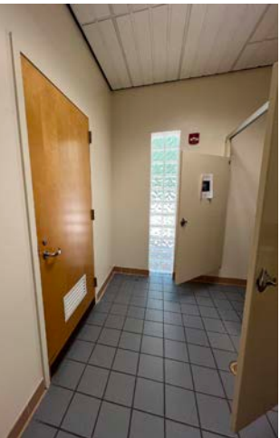
2B The door to the ADA stall should have a self-closing door
