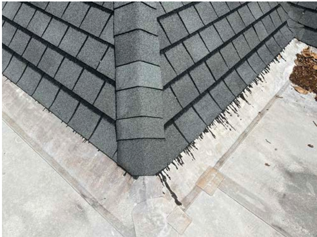
10A Interior side of shingle parapet; no termination flashing was used between the PVC roofing membrane and the asphalt shingles
