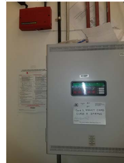
Figure 11: Fire Alarm Panel
