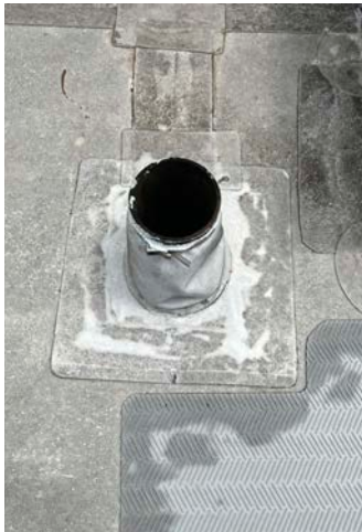
10B Roof vent condition; no leaks have been reported
