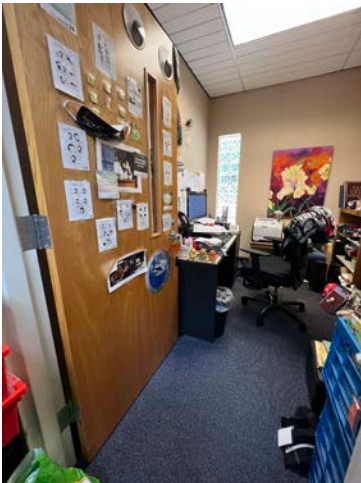
8 Current furniture arrangement impedes code required door clearance
