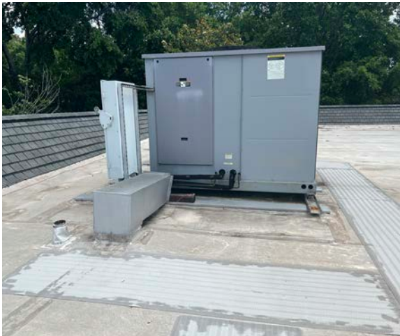
10B PVC roofing is in average condition
