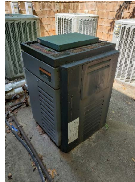
Figure 2: Hot Water Boiler
