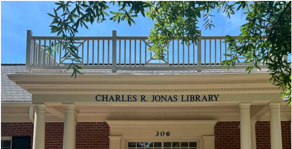
14 Railing at portico along W Main St is a maintenance nuisance; the railing is in constant need of cleaning, painting, and debris removal
