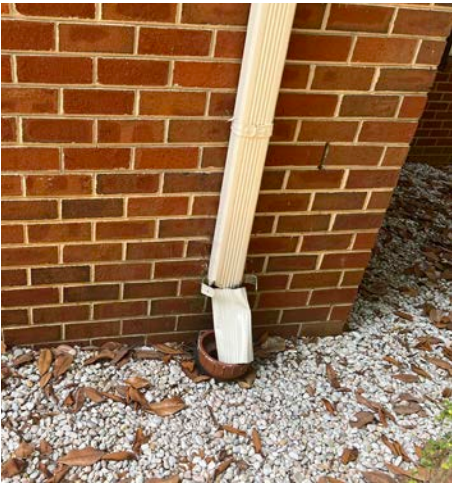
12 Some gutter to storm water connections are damaged and need replaced
