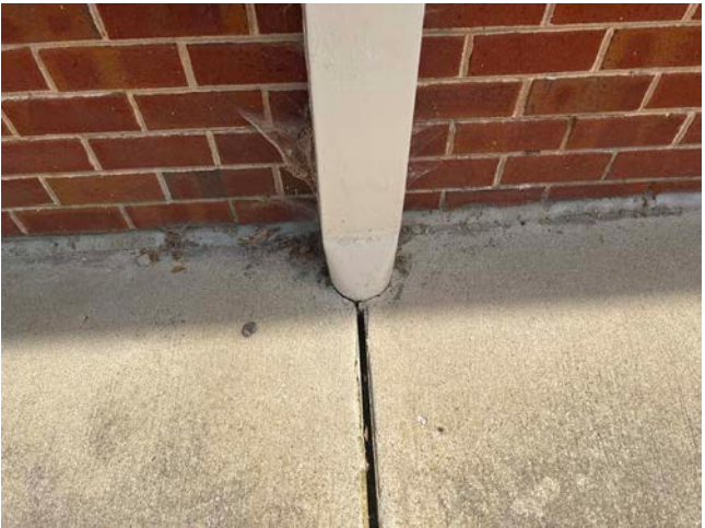
2 Heavy caulking joints are present at the sidewalk; photo taken at north side of building at the parking lot
