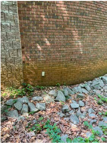
6C No flashing or weep holes are present on the northern facade of the building
