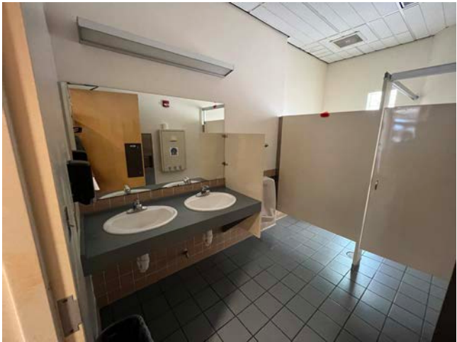
1A There are exposed pipes below the sink 1B Clear space required at sink is interrupted by the restroom door
