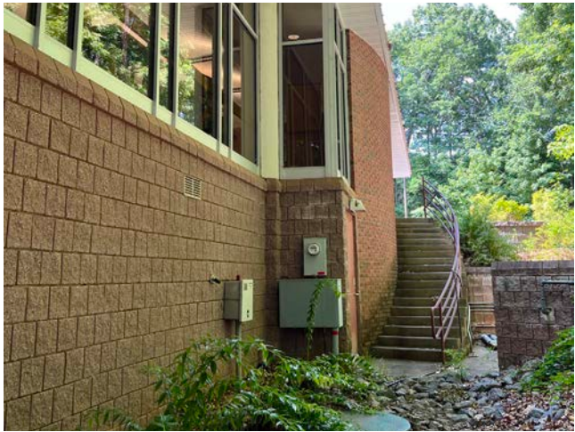
11 A railing should be installed on the face of the building to comply with current building codes; the existing stair railing could use a fresh coat of paint
