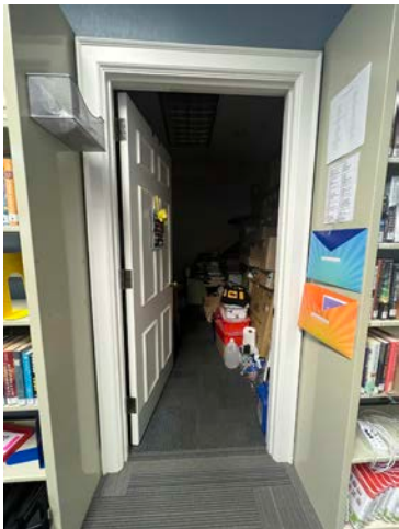
29A The office door does not have adequate clearances or room for signage
