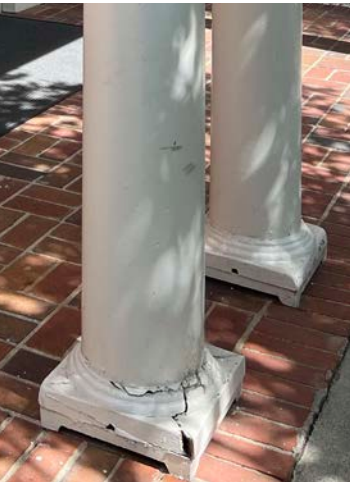
14 The column covers at the western entrance are cracked and need replaced
