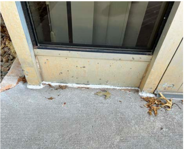
3B Storefront sill at the multipurpose room shows evidence of a prior leak; it appears leak was fixed with caulking
