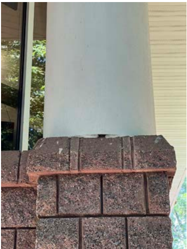
3A Caulking at the north east exterior column needs repaired
