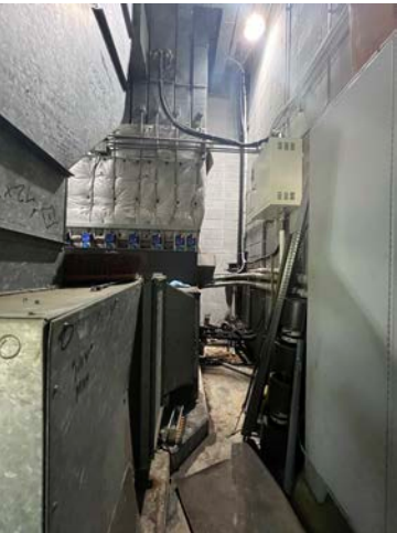
6 Mechanical room; air handler
