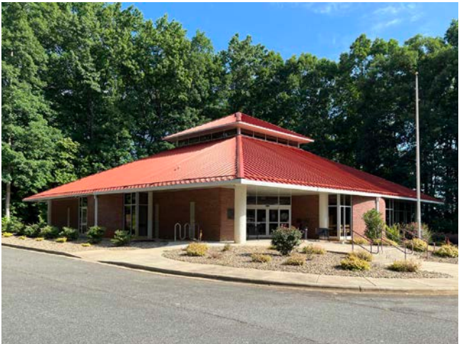
12 13A Standing seam metal roof appears to be in good condition; gutters and downspouts are provided near the entry
