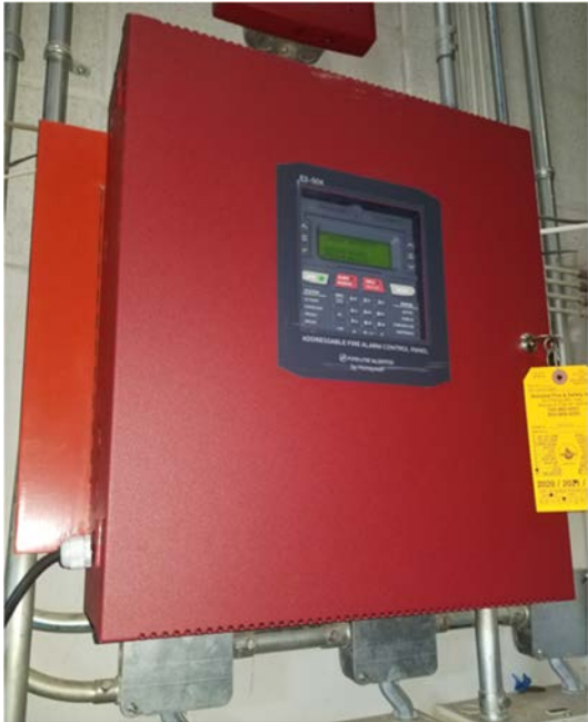
Figure 10: Fire Alarm Panel
