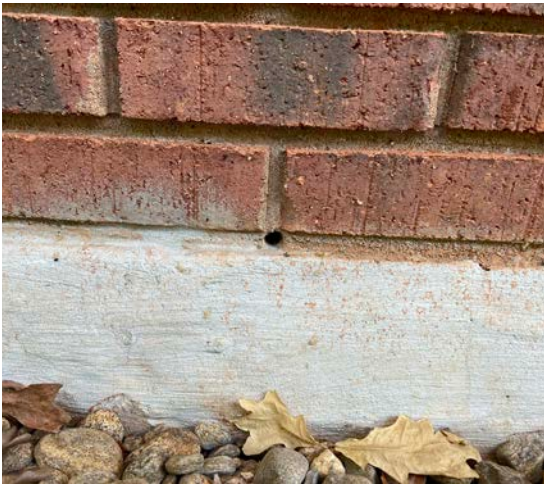
6C No flashing is provided above grade; weep holes appear to be installed post-construction in an attempt to vent the wall cavity
