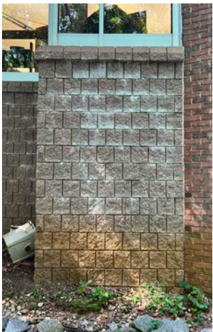
2C Brick and split face CMU are in need of a good cleaning
