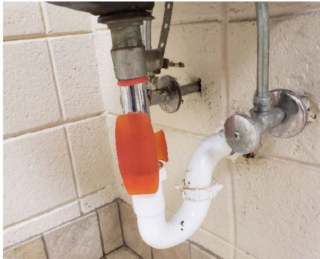
Figure 15: P-Traps
