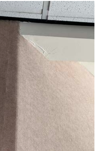
4C Water damage at soffit
