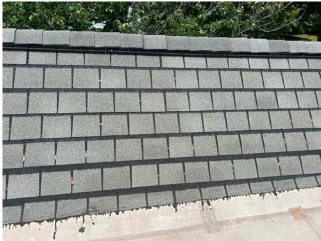
10A Interior side of shingle parapet; improper shingle overlap; roof ridge vent is in good condition
