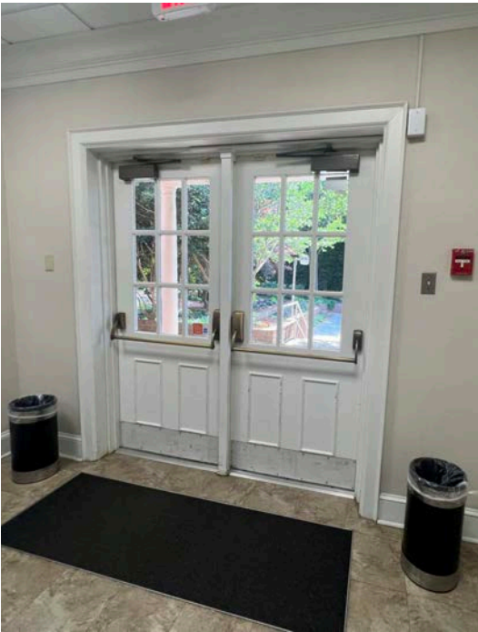
1B Non-ADA compliant push hardware on entrance
