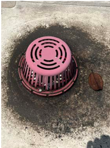
11 Roof drains appear to be functioning correctly
