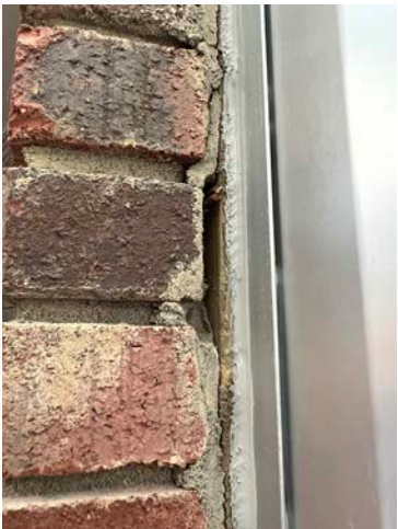
8C Wood blocking is visible at storefront jamba
