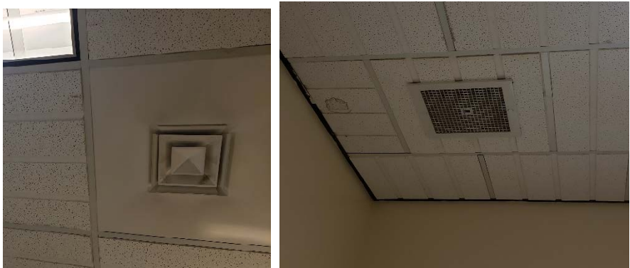
Figure 6: Diffusers (Typical)
