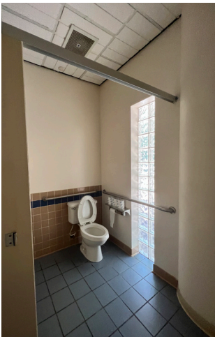
1C No vertical grab bar 1D Inadequate ADA toilet partition dimensions
