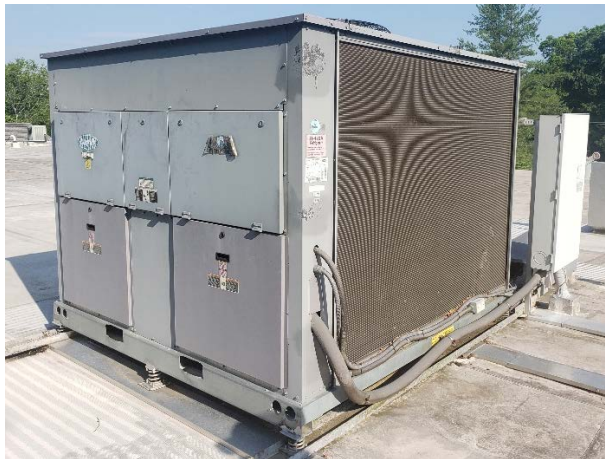
Air Cooled Condensing Unit
