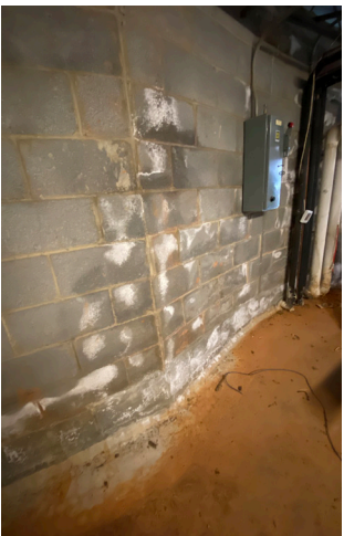
2A Efflorescence on mechanical room wall
