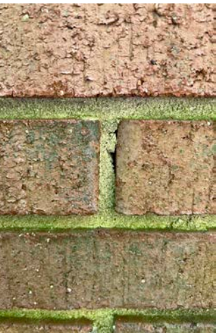
2B Raked mortar joint with moss growth; rake joint creates a ledge that holds water
