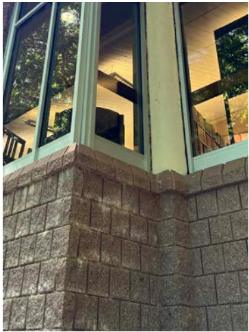
6D No flashing or weep holes are present at the sill detailing of the storefront
