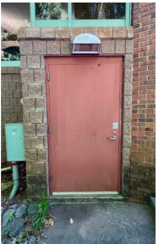
2A Efflorescence at the mechanical room door
