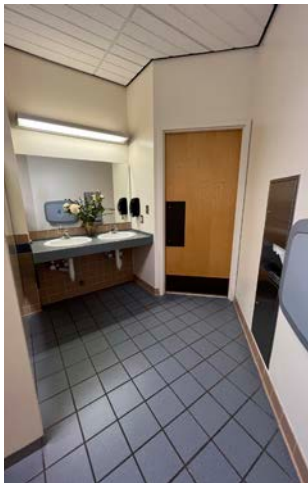
2A Exposed pipes at sink 2C Inadequate door clearance
