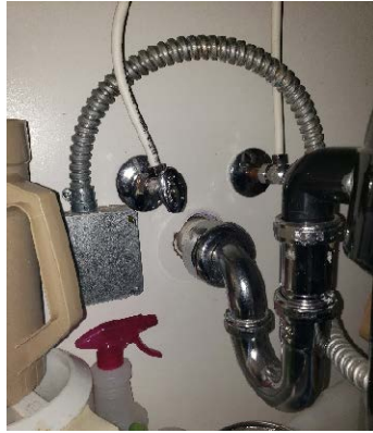
Figure 18: P-Traps
