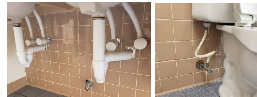
Figure 17: Sanitary Waste Line
