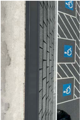
12 Gutter guards frequently get clogged with tree debris and need cleaned out
