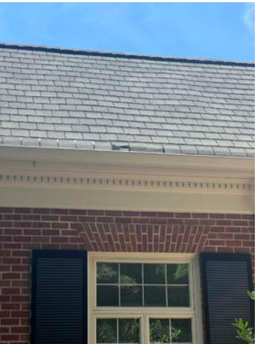
10A Incorrectly installed starter shingles; shingles often peel away at the edge condition
