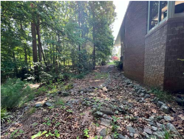
6A The trees at the north and north east side of the building make it difficult for the ground to dry out after it rains / snows.
