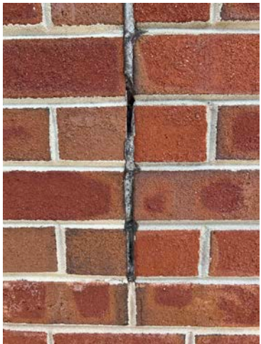
3 Control joints need replaced
