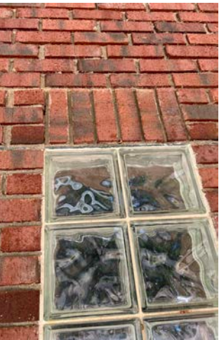
6B No flashing is present at the head detailing at the glass block
