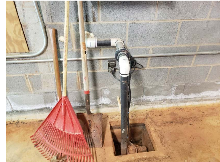
Figure 16: Sump Pump
